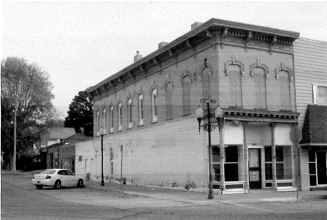
Figure 6 The 1876-1877 Star Drug Store (129 4 th St. W.) is a corner building with both elevation cornices intact as well as several original chimneys. Tallgrass Historians LC, 2015
