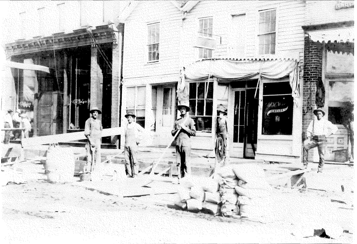
Circa 1900-1906 photo showing construction of the sidewalk along the north side of 4 th Street W. The white frame buildings in the center were replaced by 1907 with the present building (115 4 th St. W., noncontributing). The handle of A.T. Nelson's axe sign is visible on the far left edge. The cast iron columns of Nelson's storefront are extant and the modern cladding is scheduled to be removed. The picture-frame millwork door behind the man on the far right, standing with his hand on his hip, is extant also (109 4 th St. W., Downer & Derby Furniture and Hardware store).
