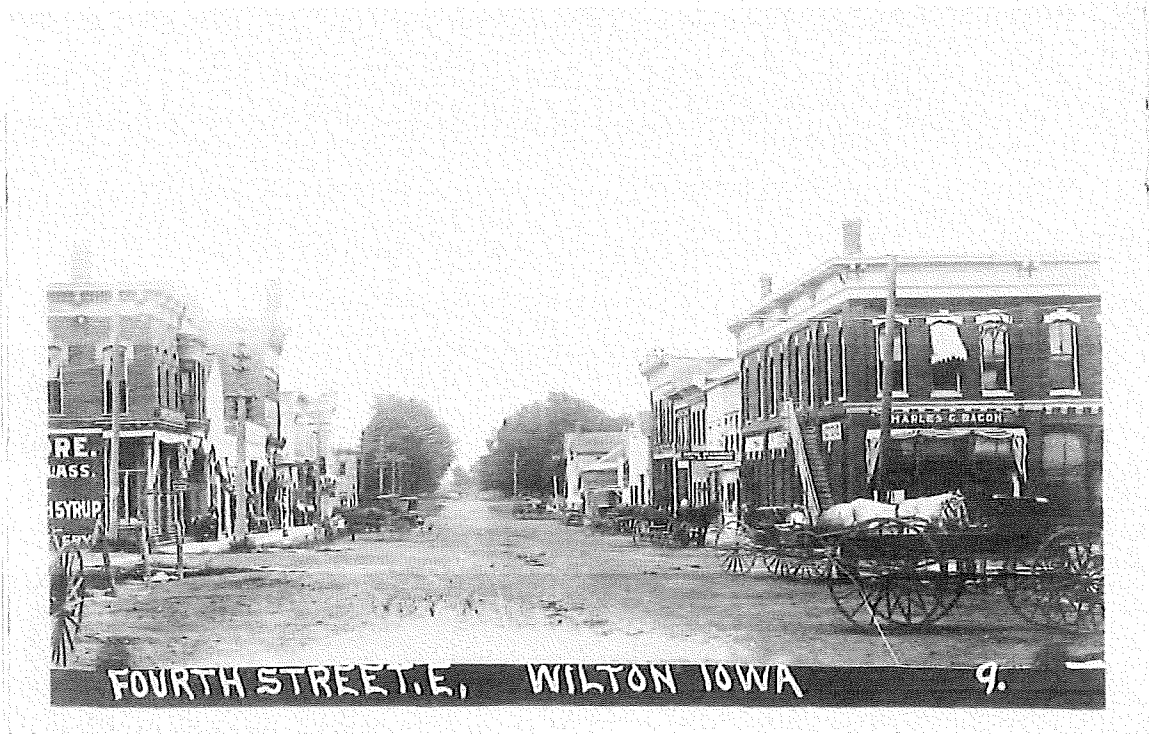
Figure 18 Commercial district streets were wide to accommodate horse-drawn wagons but left muddy after a heavy rain. These streets would not be paved until 1926. In this undated, but c. 1900 view, Star Drug is seen here on the near left edge, with the tall Scott and Johnson/opera house building a few doors down. On the opposite side of the street, the near corner building is the Bacon block, while at the end of the block in the distance, the other tall building is Fred Maurer's mercantile store. These buildings are all extant, as are most of the smaller buildings in between the brick blocks, especially on the right (south) side. Many of these smaller buildings now have poor integrity however. Provided by the Wilton Development Corporation
