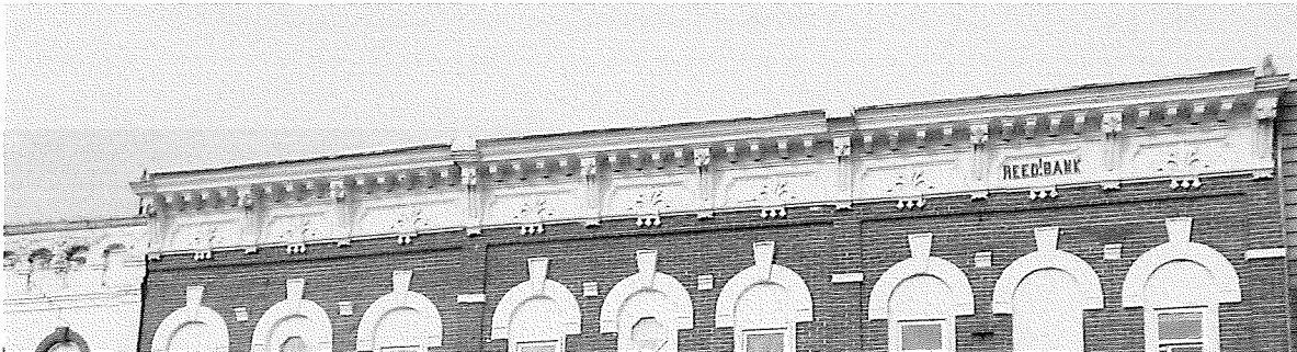
Figure 8 The south three bays of the Reed Building(313-315-317 Cedar St.) also have pressed metal cornices . Tallgrass Historians LC, 2015
