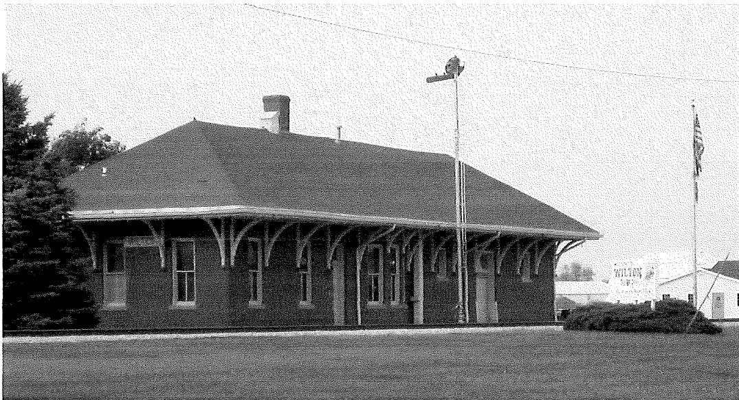
Figure 20 The Rock Island depot in Wilton is listed in the National Register of Historic Places. It is the only building in the historic district that is south of the one remaining (but still active) set of tracks. Tallgrass Historians LC, 2015
