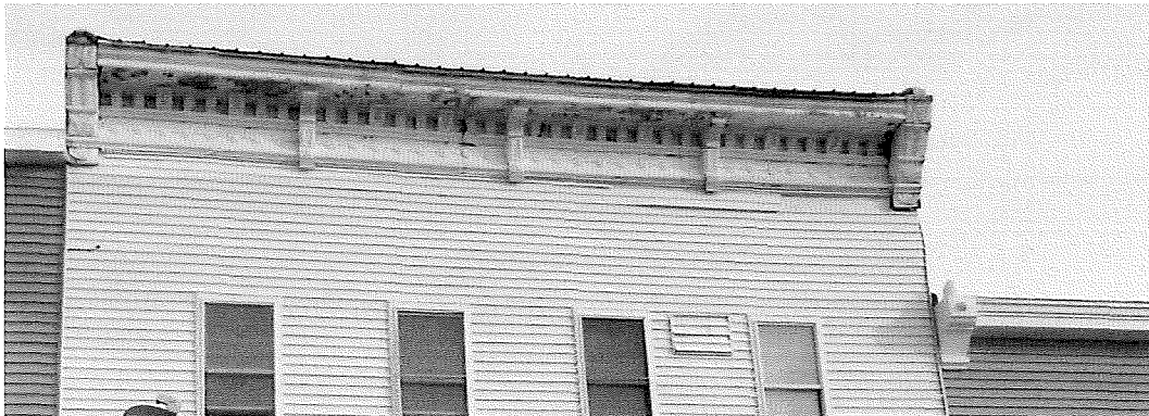
Figure 7 The turn-of-the-century Downer & Derby store building's ornate cornice (109 4 th St. W.) is pressed metal that is showing some rust. Tallgrass Historians LC, 2015
