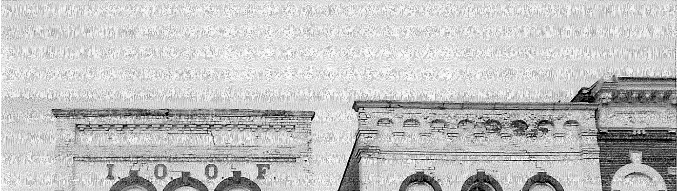
Figure 10 The Baerwald Harness Shop/IOOF hall (309 Cedar St.) and its neighbor (311 Cedar St.) have well-detailed brick cornices. The IOOF cornice is a framed corbel or mousetooth design, while the other building on the right exhibits an arcade pattern that is classically inspired. These two buildings were built soon after the 1874 fire that destroyed this block. Tallgrass Historians LC, 2015
