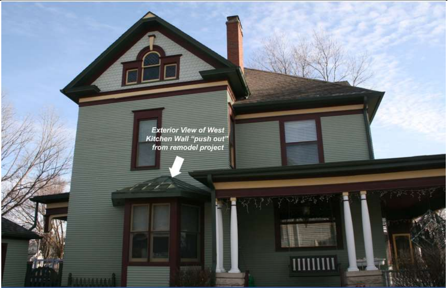
Figure 3: Photograph taken by owner Ted Marolf of renovation 8-12-19.
