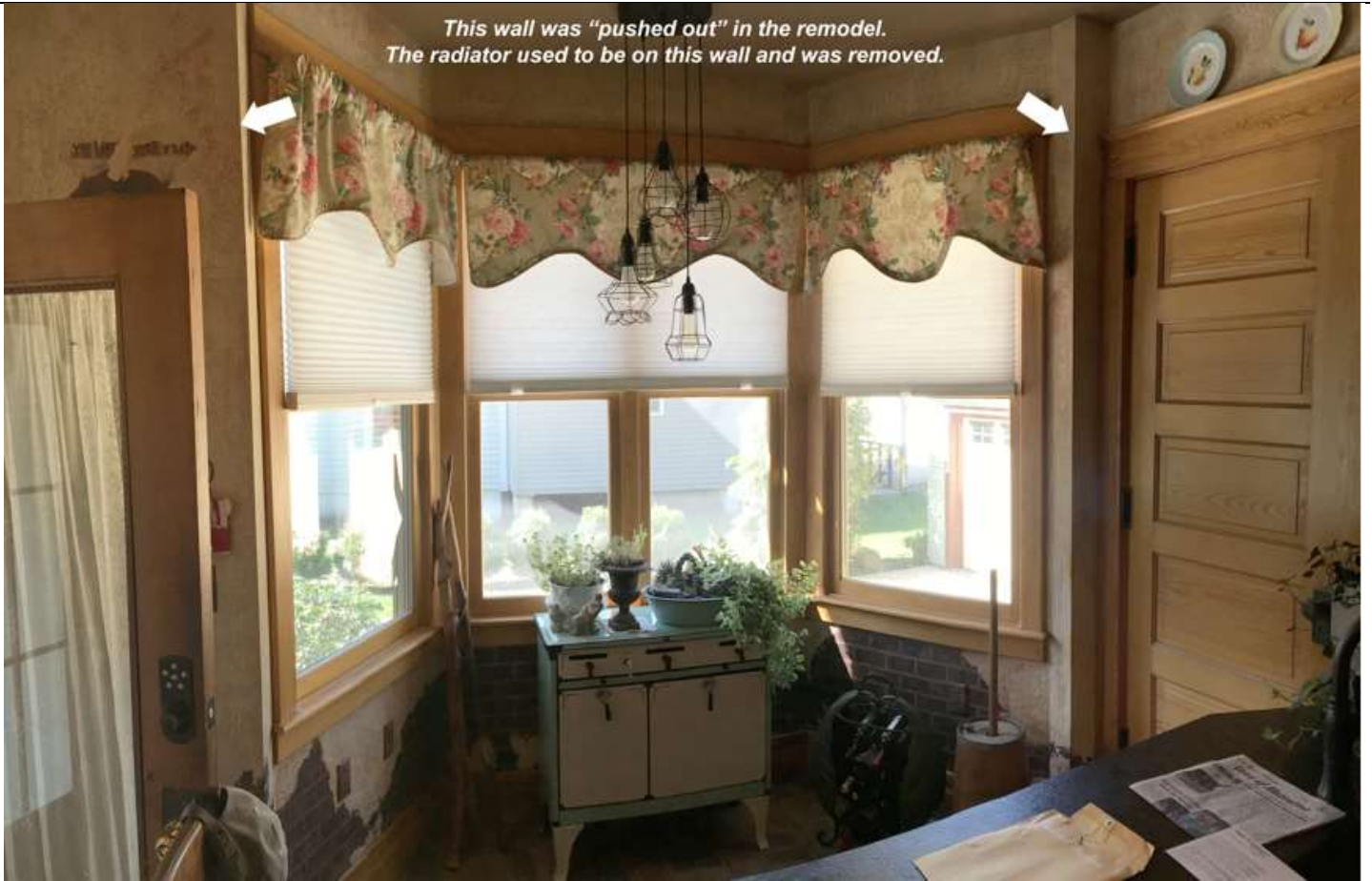
Figure 1: Photograph of the west wall of the kitchen which was punched out to install a bay window. Photo taken by owner Ted Marolf 8-12-19.
