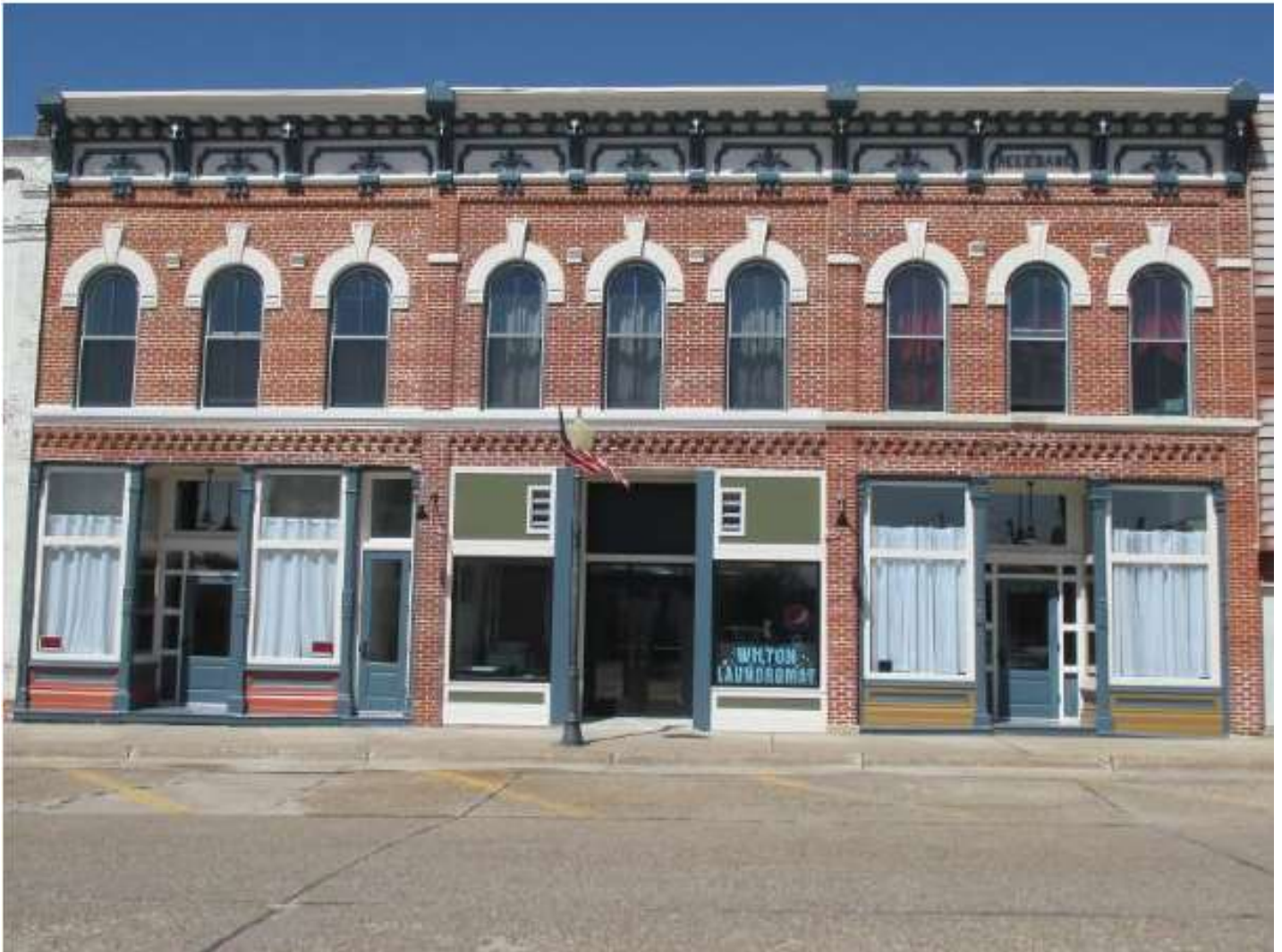
Figure 12: Picture is the Leith Commercial Building on Cedar Street in downtown Wilton in 2019. This building was recently rehabilitated with the help of a Community Development Block Grant. Photograph taken by Rebeckah Allgood 8-12-19.
