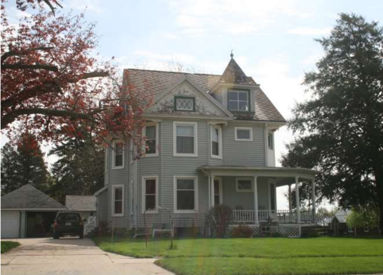
Figure 5: The Wacker House at 704 Maurer Street was built circa 1907 by John Wacker has been sided over original cedar siding and replacement windows but has some of the original wood details on dormers. John Wacker was a downtown commercial business owner. Photograph taken 8-12-19.
